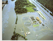
Upper Brays Bayou, Houston, TX Wastewater Treatment Plant inundation during Tropical Storm Allison, June 9 2001
