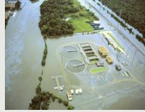
Upper Brays Bayou, Houston, TX Wastewater Treatment Plant inundation during Tropical Storm Allison, June 9 2001
