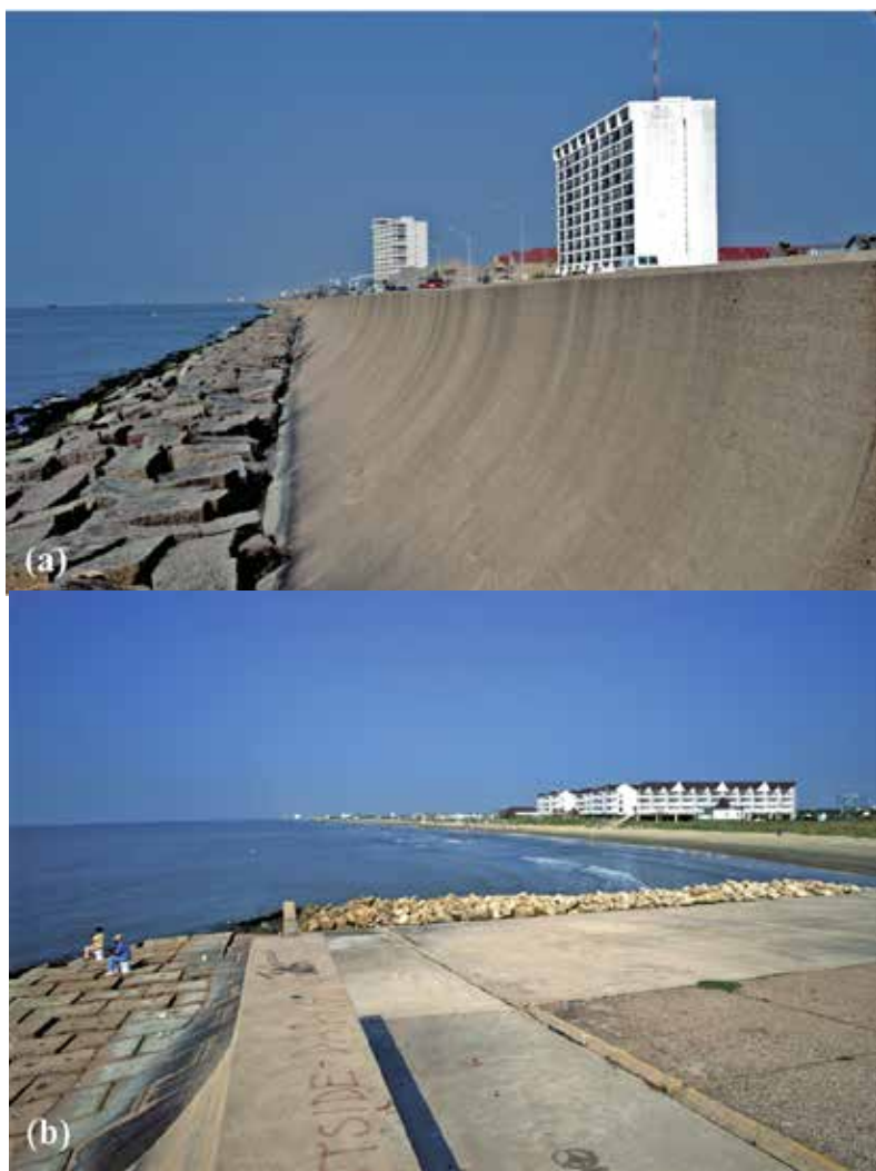
FIGURE 11-23. Seawalls are designed to protect beachfront property from erosion. (a) The Galveston seawall was constructed after the destructive hurricane of 1900. Since the wall was completed in 1962, the beach has eroded along much of its length, leaving the shoreline more exposed to attack by the highest waves of future hurricanes. (b) The barrier island has continued to retreat since the Galveston seawall was constructed. The beach just beyond the end of the wall has now retreated substantially farther shoreward than the wall's location as a result of the natural process of barrier island retreat and the consequent reduction in the amount of sand in the littoral drift system that occurred once the beach had been eroded away in front of the wall. (c) Seawalls are undermined from the sides and eventually destroyed as sea level rises.
