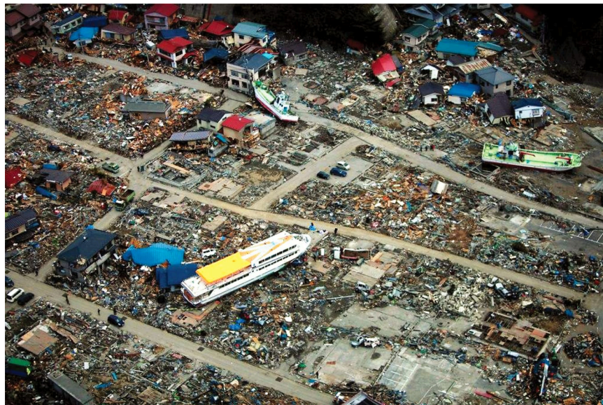
Figure 9-1. A large ferry boat rests inland amidst destroyed houses in Miyako, Iwate, Japan. The houses were destroyed and the ferryboat and other boats carried inland by a tsunami that followed a 9.0 magnitude earthquake on 11 March 2011. The earthquake and tsunami killed about 27,000 people, most of whom survived the earthquake only to be overcome by the tsunami.
