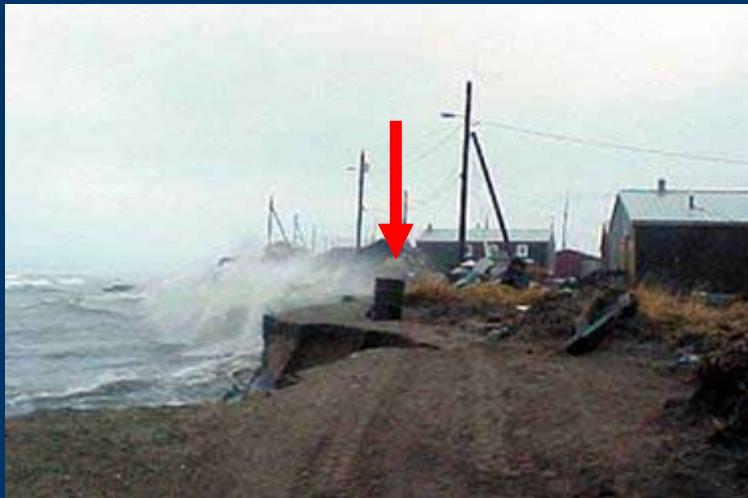
Two-hour time lapse showing storm damage Shismaref, Alaska
