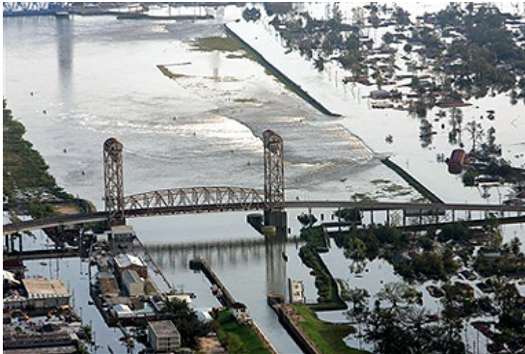
A breached levee in New Orleans, LA, after Hurricane Katrina.
