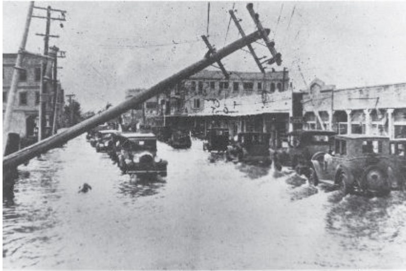
FIG. 2. Famous street scene at 12th Avenue and W. Flagler Street, Miami, after the “Miami” Hurricane of 1926 (from the Historical Association of Southern Florida).
