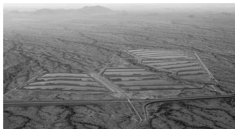
The Tonopah recharge facility takes advantage of the porous ground of the west Salt River Valley basin
